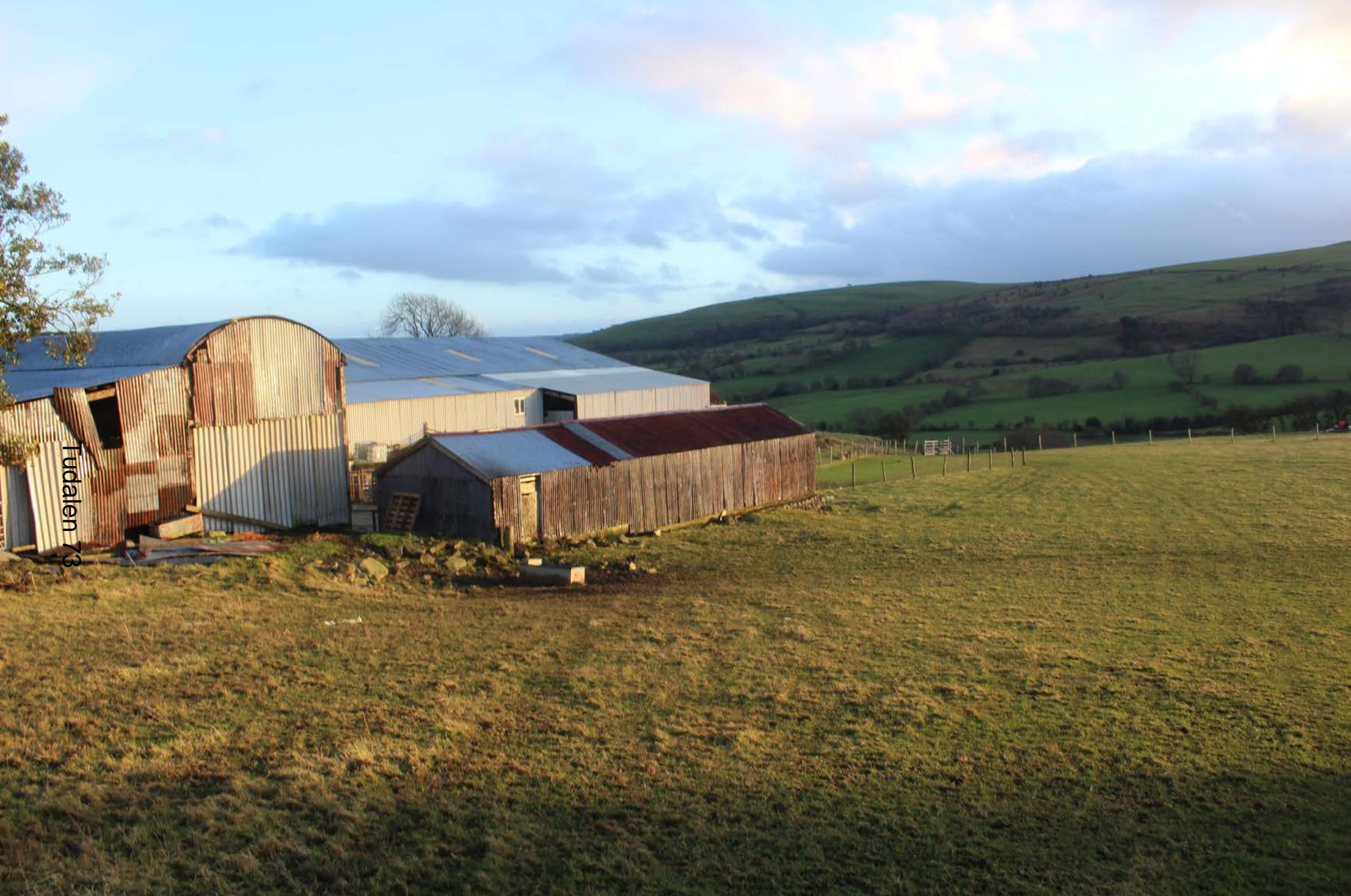
10. Site area. Please note, the units will be significantly smaller than the existing farm buildings. Also, the nearest pod will be located 97m away from the main road.
